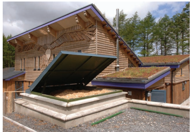
Figure 6 Fuel store for wood chips close to boiler house (Forestry Commission).
